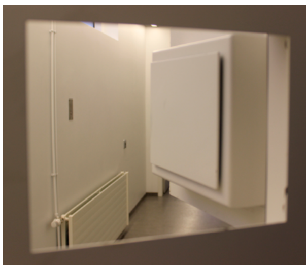
View through the hatch in the solitary confinement cells at Hólmsheiði Prison.
